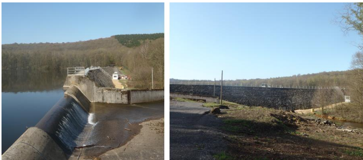
Figure 9: Barrage (source : IRH 2010)
