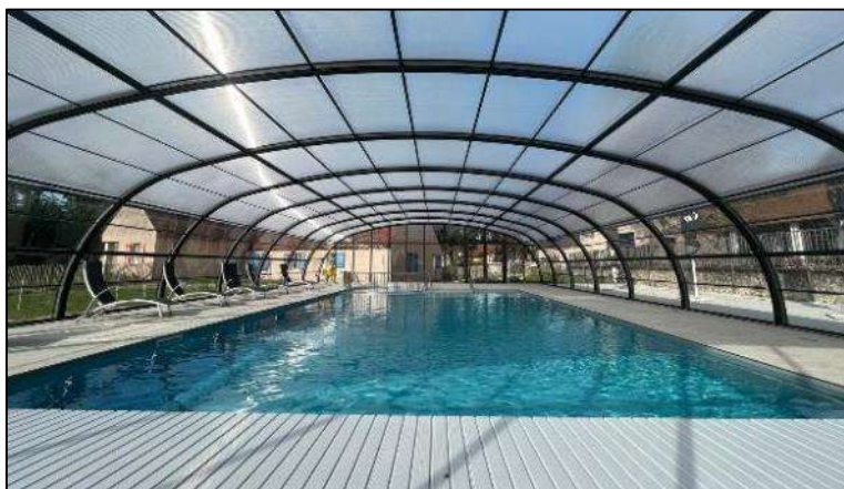
Figure 25 : Piscine attenante au camping et village vacances ( http://www.village-vacances-bellebouche.com )
